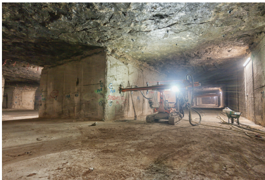
Fig. 8. Whitbed and Roach pillars have rib support put into them with the aim of preserving the pillar's cross-sectional area.
