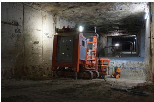
Fig. 9. Access to the Basebed is by means of two easily navigable 10° ramps which were cut into the floor of the initial Whitbed and Roach workings.
