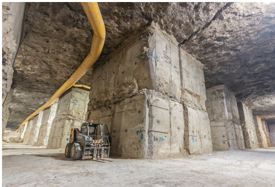
Fig. 15. The mine is force-ventilated via an 800 mm diameter pipe with smaller diameter capillary tubes feeding blind headings.
