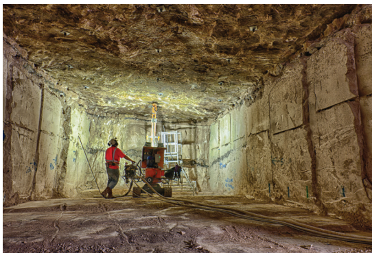
Fig. 7. The mine's roof is systematically supported using rockbolts, installed in a regular pattern which is extended up to working faces as the mine advances. All cutting operations are therefore undertaken beneath a fully supported roof-beam.
