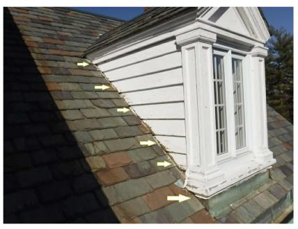
Copper flashings installed at each course of slate turn up and go behind the siding.
