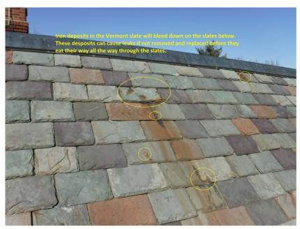
One or two of these iron deposits can cause a lot of staining.
