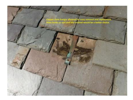
Here we can see the copper hanger that was installed to hold the replacement slate in place. While these hangers are not the best method for replacing damaged slates, it does allow for easy removal to view the fasteners.
