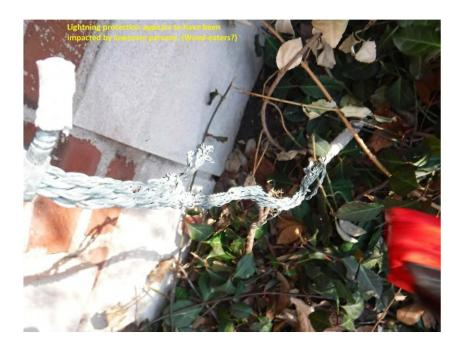
Lightning protection appears to have been damaged
