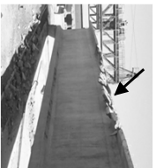
CRANE BRAKE FAILED + DROPPED SPREADER BEAM ON GIRDER
