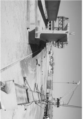
CRANE BRAKE FAILED + DROPPED SPREADER BEAM ON GIRDER
