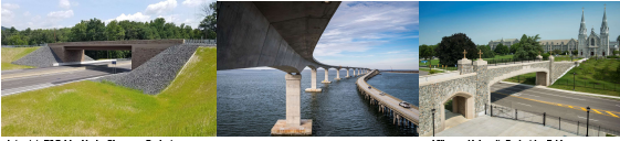
Interstate 78 Bridge Under Clearance Project Berks County, PA Macro Beam Bridge Placement of the Herbert C. Boren Bridge | Dare County, NC Villanova University Pedestrian Bridge Wayne, PA
