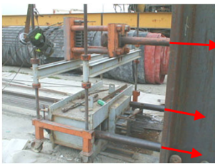
Stressing rams behind the abutments pull large rods to stress strands
