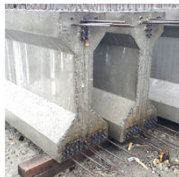
Strands burned off with short projections on ends cast into diaphragm
