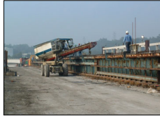
Concrete placement
