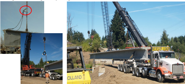
Using load triangle to pass girder between two cranes
