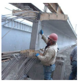
Strands burned off with short projections on ends cast into diaphragm
