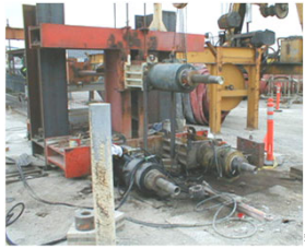
Stressing rams behind the abutments pull large rods to stress strands
