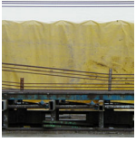
Curing tarps are used to retain heat for initial curing
