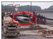
Removing retracted void form
