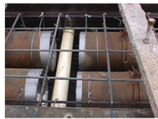
Polystyrene foam billet for trapezoidal box beam – also for conventional box beams
