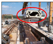
Placing expanded form for RR box beam
