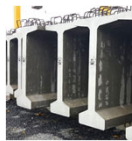
Strands cut flush & sealed on ends at expansion joints
