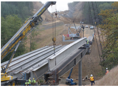
Two cranes lift girder while dollies are repositioned
