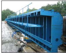
Girder side forms
