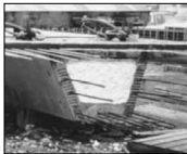
Polystyrene foam billet for trapezoidal box beam – also for conventional box beams
