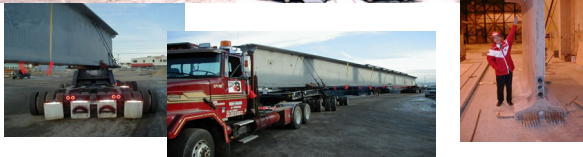
210 ft long single-piece girder - NU 2800 (110 in.)
