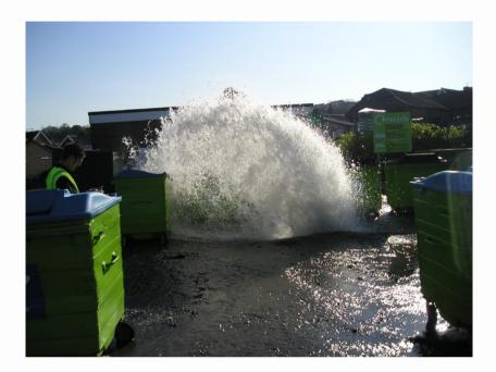
Decreasing the cover over our mains can cause them to fail, especially if vehicles are subsequently driven over them. Increasing the cover over our mains can cause difficulties when we need to repair or maintain them, as deeper excavations will be required.
