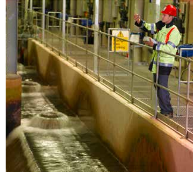
Barrow Treatment Plant
