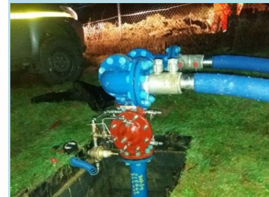
The overland solution, bypassing the burst pipe
