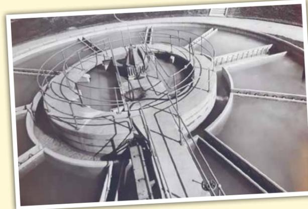
While amalgamating with other companies, Bristol Waterworks continued to innovate in water treatment. The Accelerator introduced at Stowey in 1954 was a state-of-the-art clarification and water softening plan.
