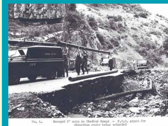
No. 4. Damaged 9" main in Cheddar Gorge - P.V.C. pipes for diversion route being unloaded
