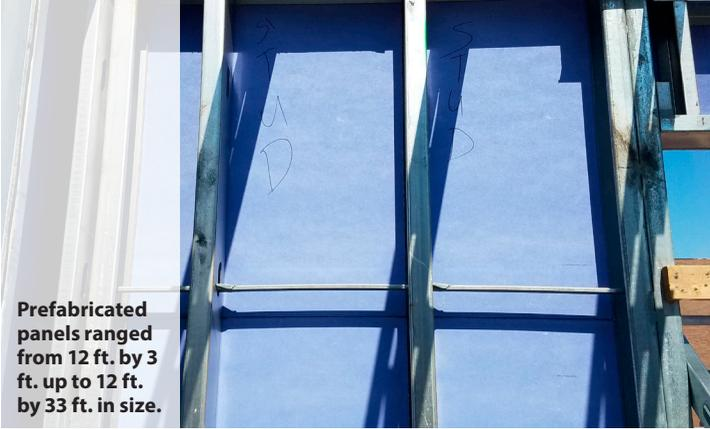
The structural system involved a hybrid of CFS load-bearing panels and bar-joist steel.
