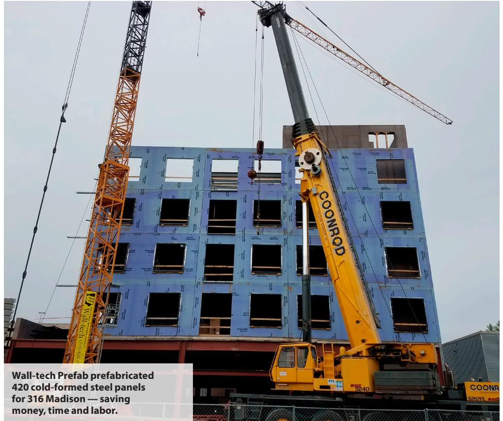
Wall-tech Prefab prefabricated 420 cold-formed steel panels for 316 Madison — saving money, time and labor.
