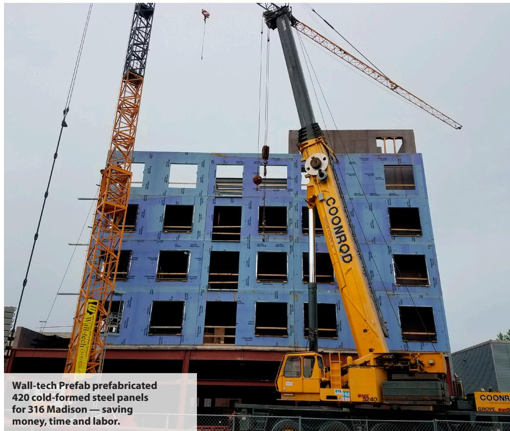
Wall-tech Prefab prefabricated 420 cold-formed steel panels for 316 Madison — saving money, time and labor.
