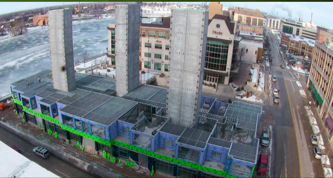
On February 1, 2016, erection of the CFS framing on the second floor of Metreau Apartments was nearly complete.
