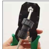
10. Insert the connector in the crimping tool and crimp to hold the wires in place
