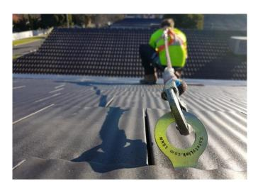
SafetyLink's team designed the TileLink roof anchor (winner of an episode on ABC1 The New Inventors) with unique energy absorbing capabilities, to reduce the risk of injury to the person and damage to the structure.
