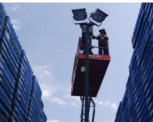
In addition to markedly reducing the lighting energy use, by installing long-lasting LED's, backed by generous 35,000 hour / 7-year warranties, CHEP has also been able to reduce its ongoing lighting maintenance requirements – costs that mount-up over time, particularly in areas that require special access equipment to reach the lights.
