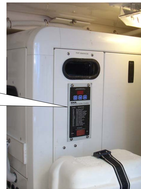
Generator control panel
