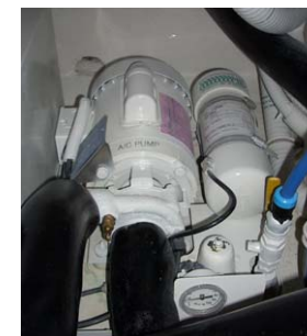
Air conditioning units and A/C pump
