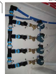
Manifolds and WC solenoid valves
