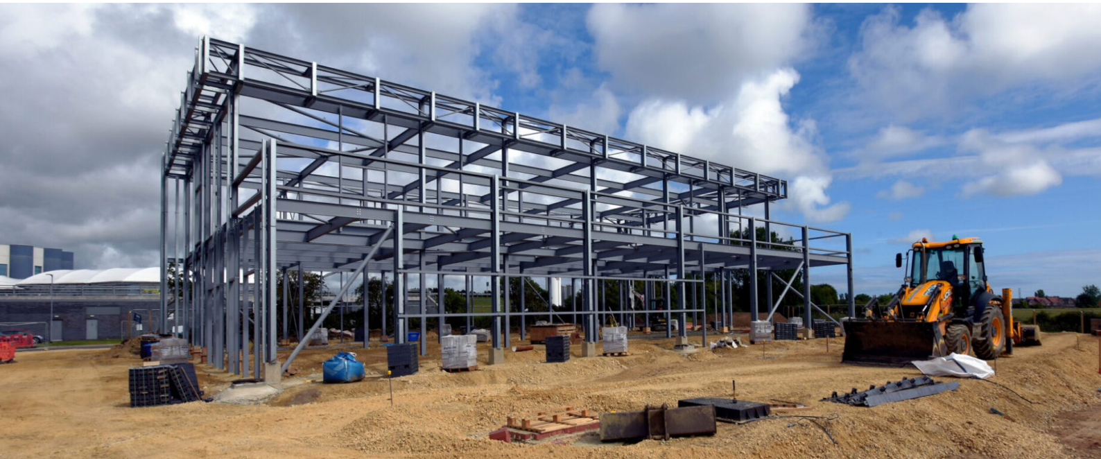
The new NHS facility under construction. Creator: Will Walker / North News Picture courtesy of North News & Pictures northnews.co.uk
