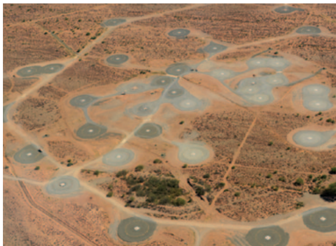
Antenna foundations in the core of the MeerKAT array, as seen in this image from February 2014.
