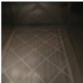
Furnace Filter Condition 09/10/2020 9:47 AM
