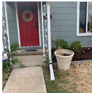
Roof / Gutters / Downspout (1/4) 09/10/2020 9:52 AM
