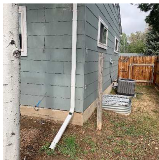
Roof / Gutters / Downspout (4/4) 09/10/2020 9:54 AM
