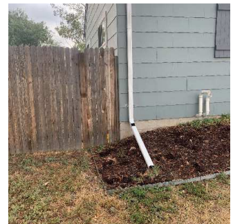
Roof / Gutters / Downspout (2/4) 09/10/2020 9:52 AM
