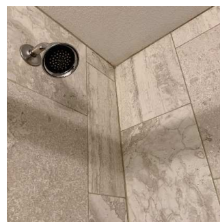
Tiles / Grout (2/3) 09/10/2020 9:42 AM
