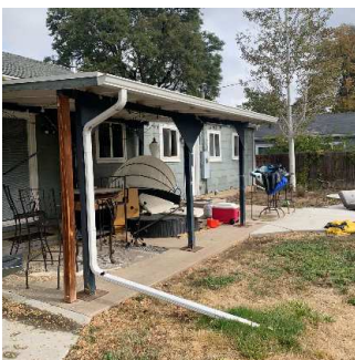
Roof / Gutters / Downspout (3/4) 09/10/2020 9:54 AM
