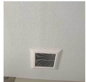
Ventilation Source (Fan) 09/10/2020 9:33 AM
