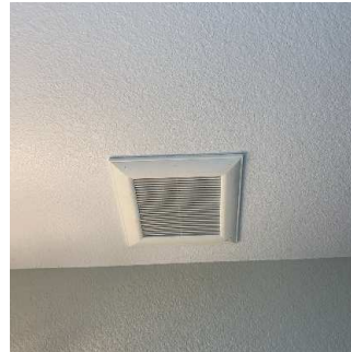
Ventilation Source (Fan) 09/10/2020 9:37 AM
