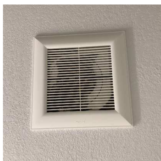
Ventilation Source (Fan) 09/10/2020 9:42 AM
