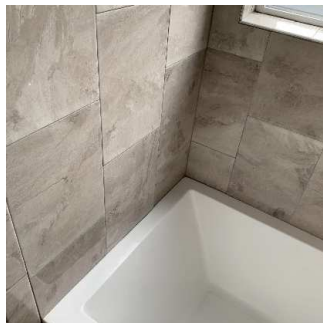
Tiles / Grout (3/4) 09/10/2020 9:33 AM
