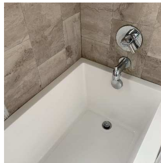
Tiles / Grout (4/4) 09/10/2020 9:33 AM
