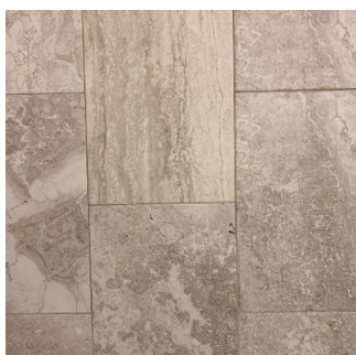
Tiles / Grout (3/3) 09/10/2020 9:42 AM
