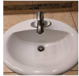
Sink & Underneath Sink (3/4) 02/02/2021 2:03 PM
