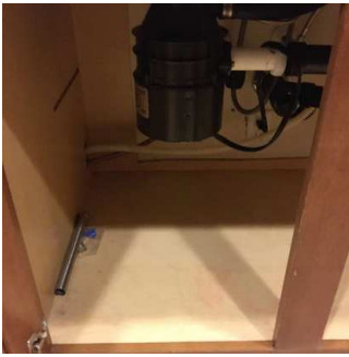
Sink & Underneath Sink (2/2) 02/02/2021 1:35 PM
