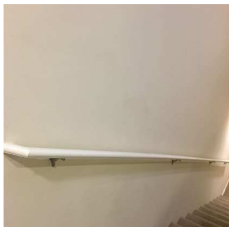
Walls & Windows (1/3) 02/02/2021 1:22 PM
