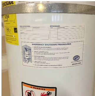
Water heater (3/5) 02/02/2021 2:12 PM
