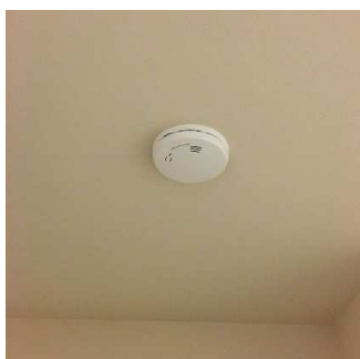
Smoke / CO detector 02/02/2021 1:55 PM
