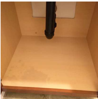
Sink & Underneath Sink (2/2) 02/02/2021 1:52 PM
