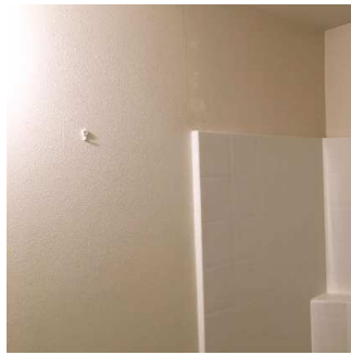
Walls & Windows (4/7) 02/02/2021 1:50 PM
