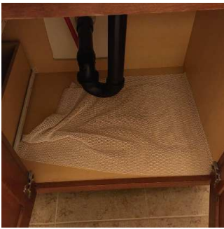
Sink & Underneath Sink (4/4) 02/02/2021 2:03 PM
