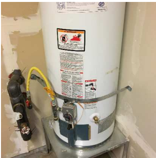
Water heater (2/5) 02/02/2021 2:12 PM
