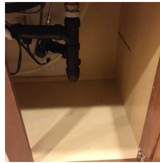
Sink & Underneath Sink (1/2) 02/02/2021 1:35 PM
