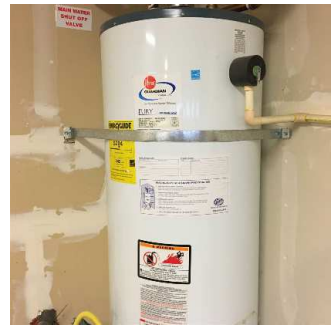
Water heater (1/5) 02/02/2021 2:12 PM
