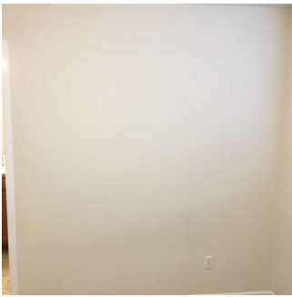
Walls & Windows (2/4) 02/02/2021 1:45 PM
