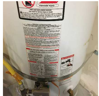
Water heater (5/5) 02/02/2021 2:12 PM
