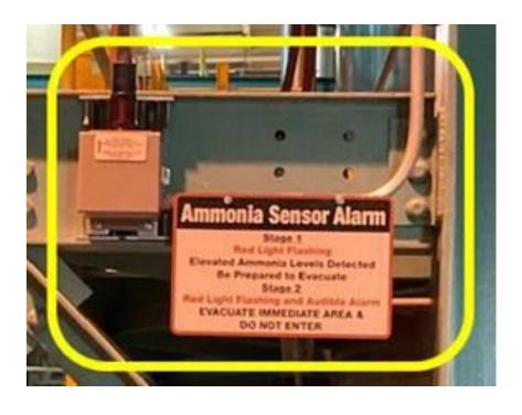
The ammonia alarm systems will monitor ammonia concentrations and alert the Operator, Boilerhouse and anybody in the kitchen of elevated levels. There are red lights and signs at every entrance to the kitchen, along with an audible alarm. The control panel is located at the coating office.
