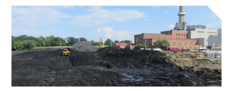
unique solution where coal ash was beneficially used as embankment fill material at the landfill. This approach demonstrated how waste coal ash could be used for an essential purpose by mitigating coal ash's unique and challenging material properties using layers of geogrid under the road base.
