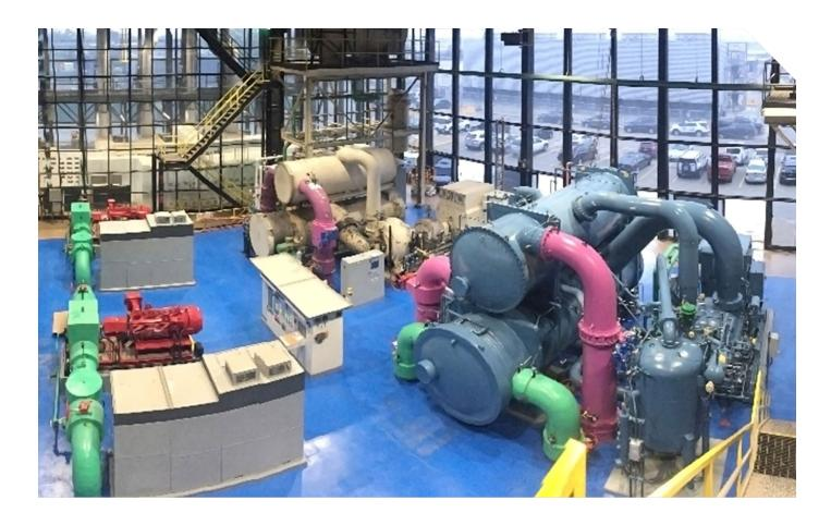
evaluated multiple options. Variable speed chillers, a combination of variable and constant speed chillers, variable speed pumps, and a thermal energy storage (TES) tank to upgrade the chilled water system were all considered. A final design was selected that included variable speed chillers and a variable primary pumping system.
