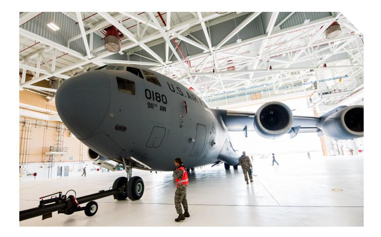
The corrosion control bay section of the hangar was designed and built to offer an environmentally controlled area to wash aircraft, provide corrosion treatment and repair, and perform aircraft maintenance painting as needed.
