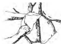
FIG. 5 GROUT JOINTS
