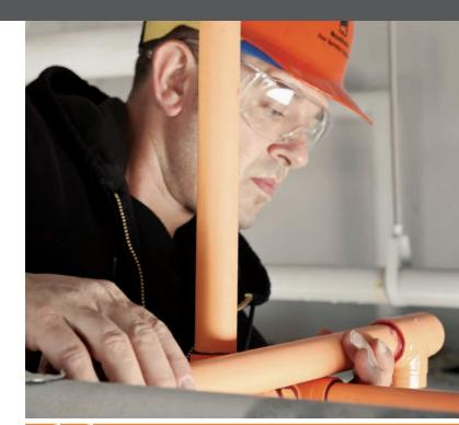
The many design alterations throughout construction made the use of BlazeMaster CPVC a more easily adaptable system than steel, which would have required refabbing in the field.
