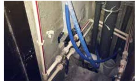
hotel guest comfort (low water pressure, water noise). These issues can be attributed to the original building system consisting of PEX and PVC pipes, which lead to poor resistance over years of use.
