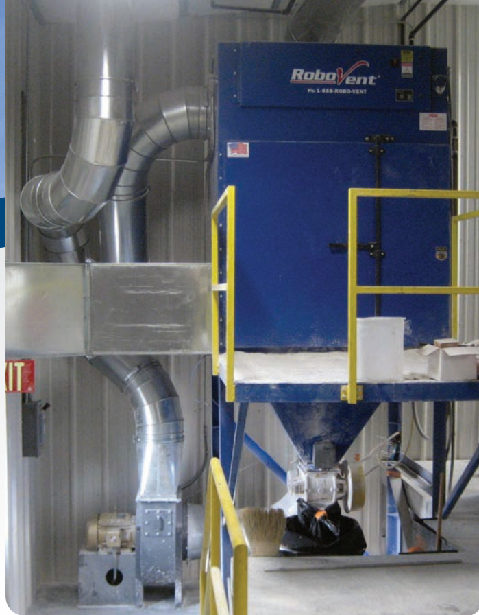
RoboVent unit collecting dust from a fiberglass sanding operation.
