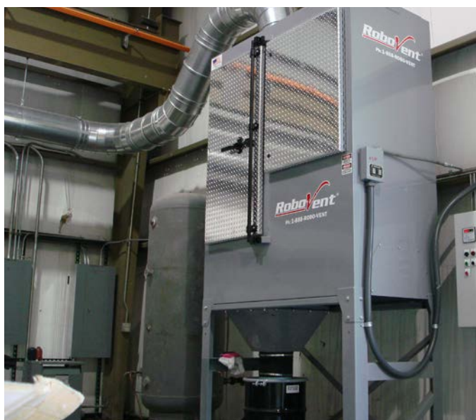
RoboVent collector used to remove dust from an industrial sandblasting application.
