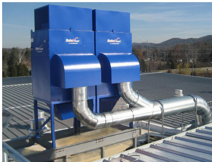
RoboVent rooftop units for a plastic cutting process.
