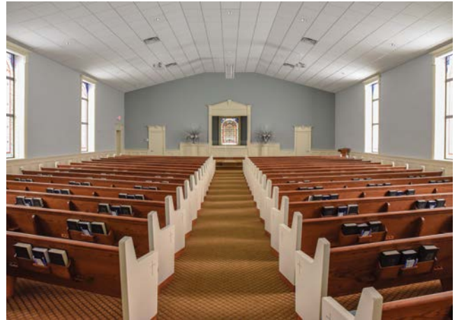
The wood-framed church required a complete overhaul, all the way down to the stained glass windows in the sanctuary.
