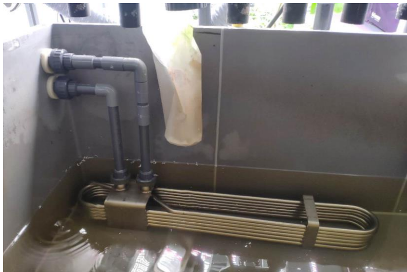
Stainless Steel Cooling Coil installed in reservoir
