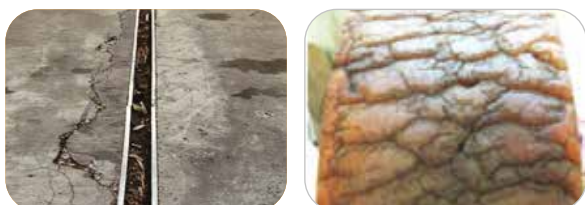
Joint deterioration
