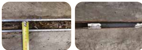
Construction or contraction joint repair
