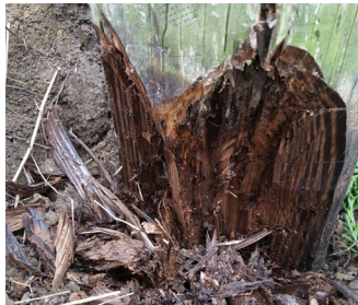
Rejected after Osmose inspection
