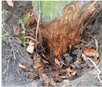
Rejected after Osmose inspection
