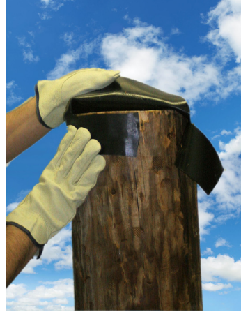
Step 3: Wrap tabs around pole and fold excess top over edges*
