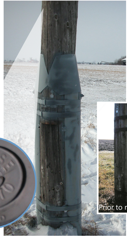
Installed in 1970; new bands and cover cap installed in 2008 - In service 47 years and counting!
