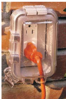
Figure 9 - In Use Weatherproof Receptacle Cover
