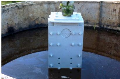
For both phases of this restoration, the foundations were cleaned and cost-effective engineered repair solutions were installed. All of the foundations then received a protective coating, and cathodic protection was installed to mitigate the on-set of further corrosion.
