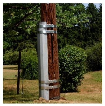
Optimized C-Truss Installed
