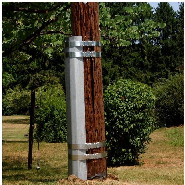
Optimized C-Truss Installed
