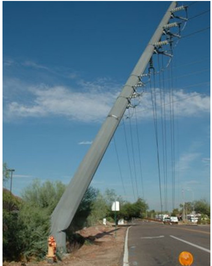
Figure 2. Steel Pole Localized Buckling Failure.
