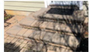
railing missing
