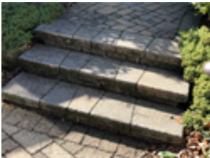
railing missing
