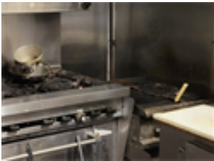
grease/debris build up
