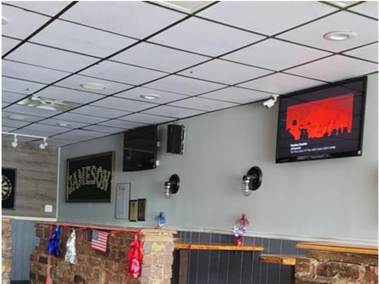
Missing Smoke Detectors
