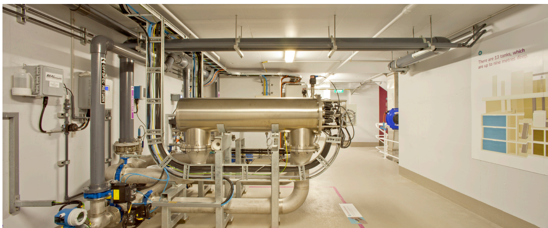
Image: Ultraviolet disinfection at Central Park Local Water Centre. Source: Flow Systems
