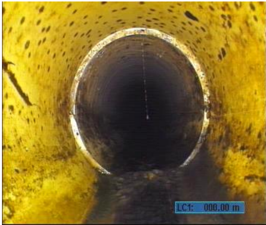
Figure 8: Example of a minor joint displacement identified by VAPAR algorithm (score = 2) but typically not reported by operators.
