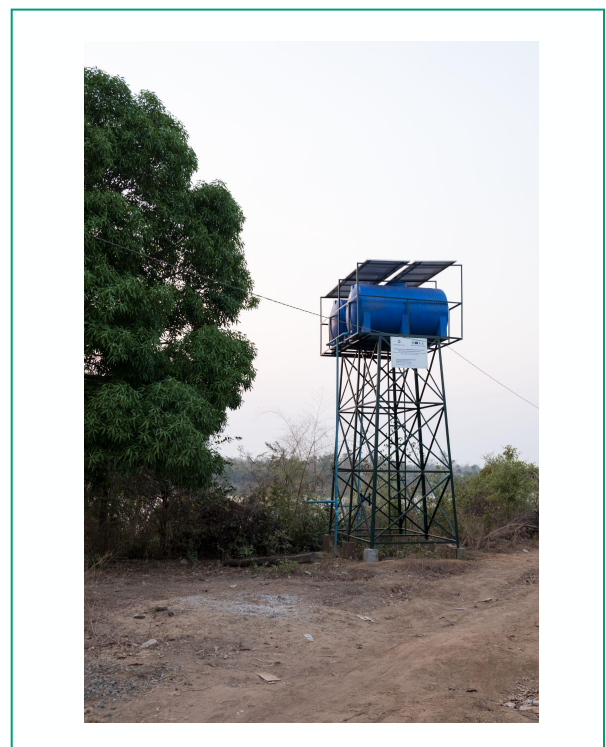
Figure 1 - Community scale water system in Ksach Leav
