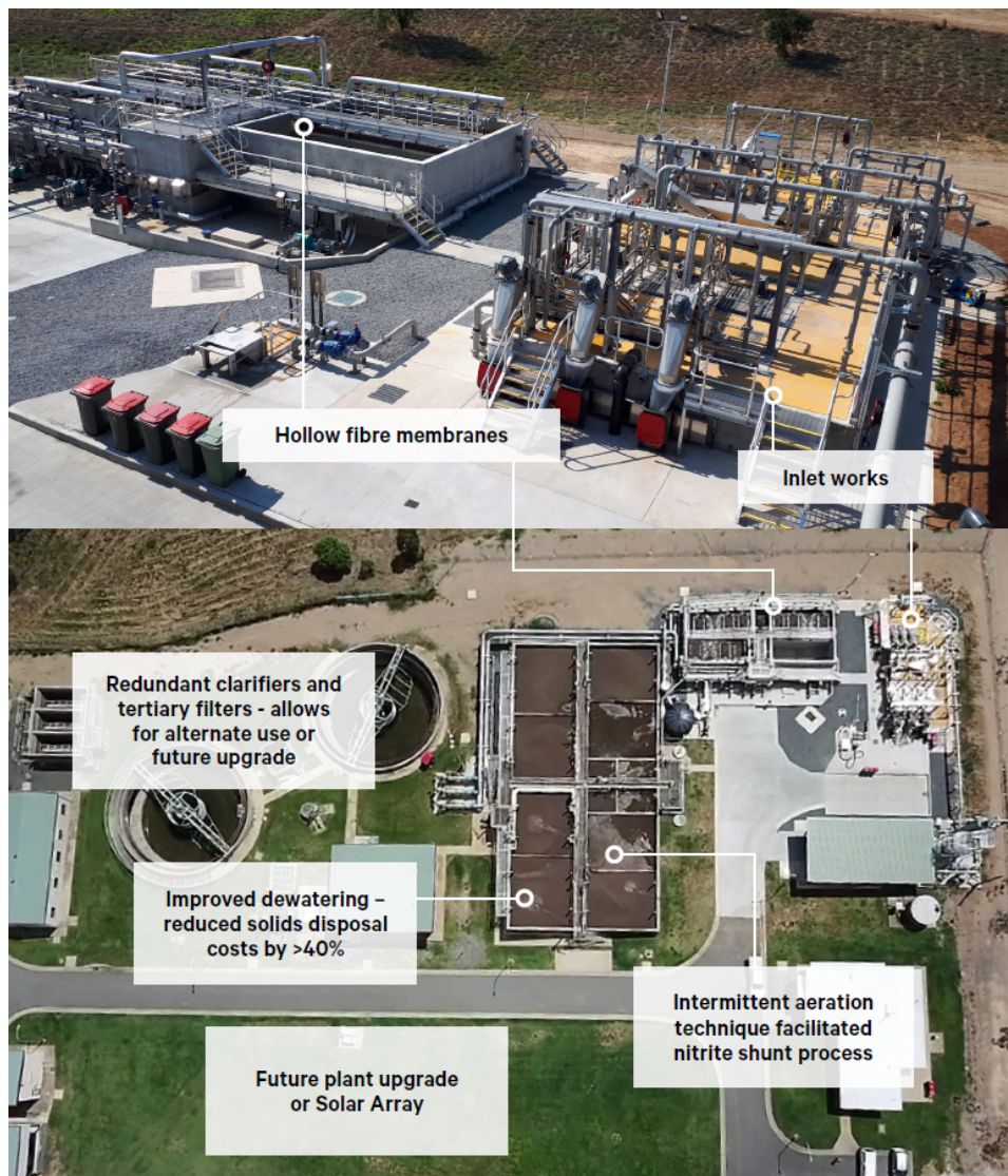
Figure 2: Aerial view of the membrane bioreactor tank and inlet works with two stage screening and grit removal (top). Aerial view of Yeppoon Sewage Treatment plant after the upgrade complete showing the footprint of the new plant is reduced, compared to the existing plant, leaving room for additional future infrastructure (bottom).
