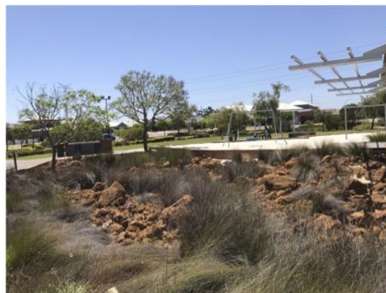
Figure 3: Sites where remediating damage caused by groundwater flooding has imposed significant costs on local government. On the left, the road intersection shown has had to be rebuilt following groundwater damage. On the right, public open space that routinely flooded with winter groundwater has been excavated and replaced by this rocky detention basin – at considerable expense, and to the detriment of the overall amenity of the green space.
