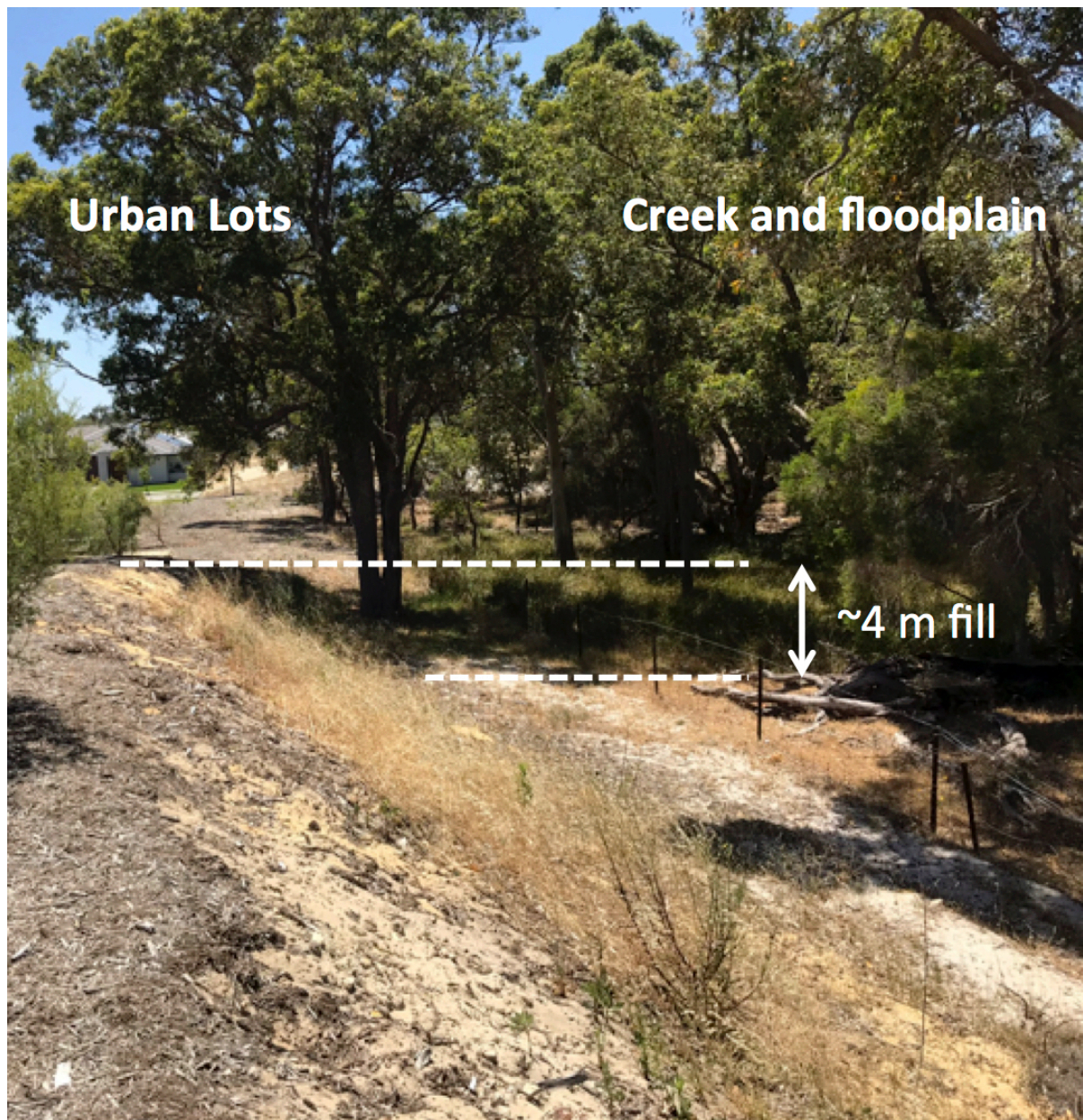
Figure 1: Illustration of extensive use of fill in a new urban development in Perth's North-Eastern Corridor. Abutting a creek, its floodplain and protected bushland, the developed land surface was elevated by as much as 4m above the natural land surface.
