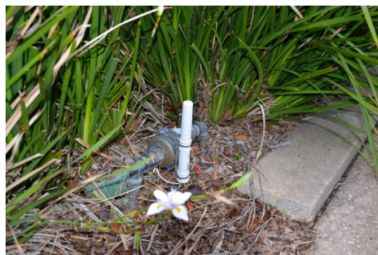
Figure 2: An example of a retro-fitted device on an existing urban meter.
