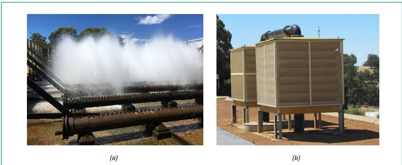
**Figure 1: (a) Spray aeration and (b) Multi-tray aerator units in groundwater treatment plants in Western Australia.**
