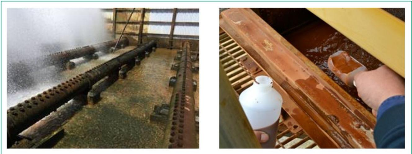
**Figure 2: Spray aeration system with slime deposits and reddish-brown deposit from tray aeration units resulting in fouling.**
