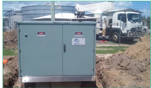
Figure 3: Installation of New 1000kVA Transformer
