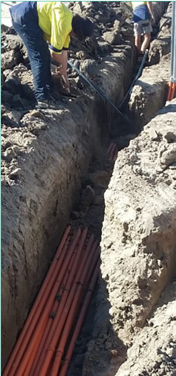
Figure 6: 25kms of DC Cable runs
