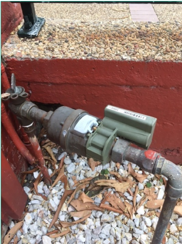
Figure 1: Residential water meter fitted with a smart water meter radio transmitter (Photo by Terry Randall)
