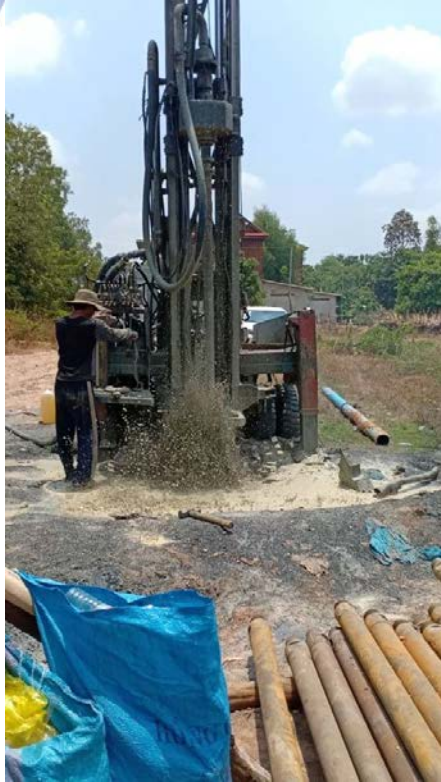
Air Rotary Drill digging 150m deep borehole (3-4 m 3 /h yield) in Cambodia
