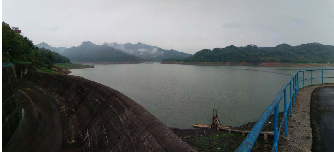
Sempor Water Reservoir providing flow rate of 120 L/s in Indonesia
