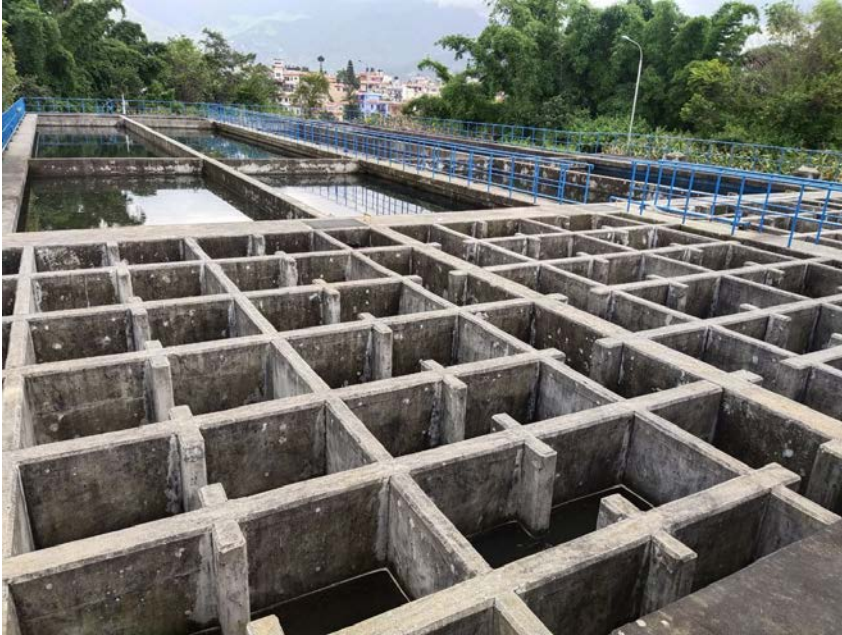
Bansbari Water Treatment Plant at Kathmandu (capacity = 21ML)
