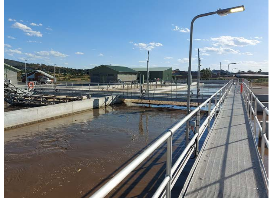
Goulburn Wastewater Treatment Plant – Membrane Bioreactor - 30,000EP
